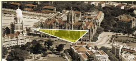
Aerial View of the Victoria terminus showing the position from where image was taken
