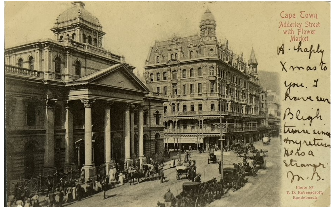
The Standard Bank building with Cartwrights Corner in the background.
