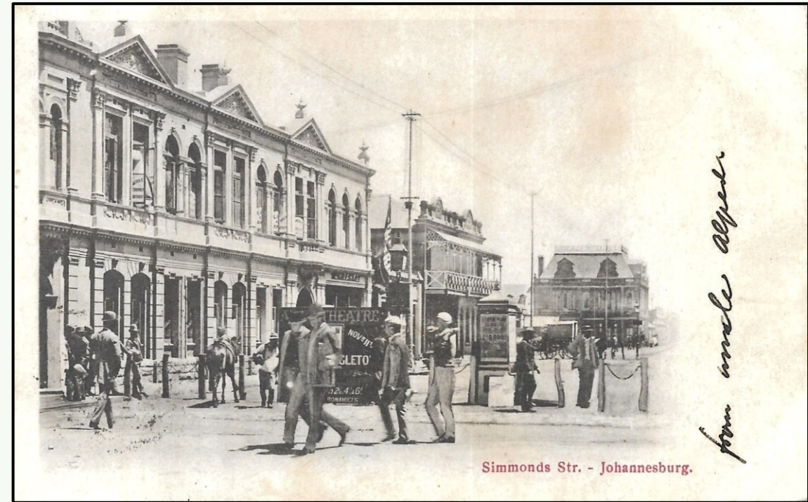
First Stock Exchange Building. To the extreme right is the Lewis and Marks building with its Hatherley Distillery sign on top
