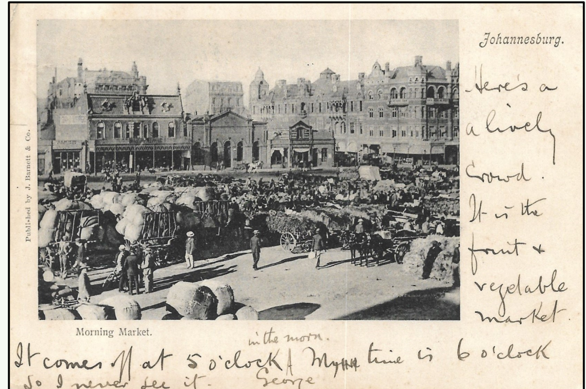
Fruit & Vegetable Market at 5 o'clock in the morning annotated in manuscript. From L to R: Birch Building (1895); First Natal Bank (1891) and the Guildhall Bar (1894) at the corner of Harrison and Market Streets. Across the road is the Steytler Building (1895) Published by J Barnett & Co, Johannesburg and UB in black
