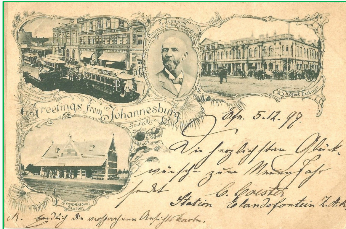
Images L to R: Commissioner Street with trams in front of Old Standard Bank (1889) and Greens Building (1894); Johannesburg Stock Exchange (1888); Below - Jeppestown Station (1896). In the middle is an image of E Hancock, a Banker and chairman of the Sanitary Board - later the City Council. Also, a founder member of the Johannesburg Stock Exchange
