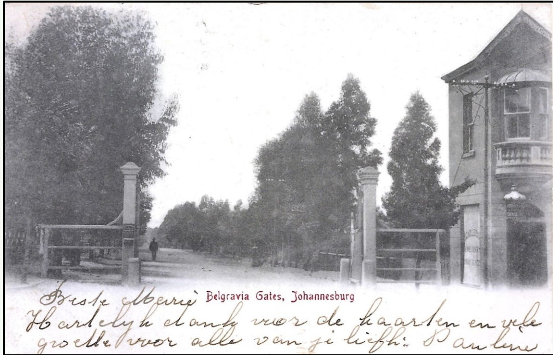
Belgravia Gates, site of early toll gates . The name J C Koller Chemist, Druggist appears in the window of the building Published by P. S. & C., Box 1205, Cape Town. Serial number 801, UB in green
