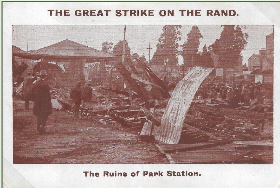
View of the ruined Railway goods shed
