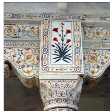
Floral motif using Pietra Dura on the pillars and walls of Taj Mahal.
